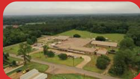
TIOGA ELEMENTARY SCHOOL
